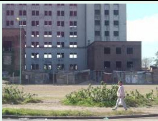
The construction of this hospital in Mataderos was abandoned decades ago. Now police patrol it around the clock to prevent the homeless from sleeping in the empty floors. The poor instead live in the cardboard houses at the foot of the hospital.
